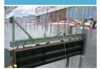
Stop logs are hydraulic steel structures for stopping the water streams of water upstream of sluices or hydroelectric power plants. They serve to shut off water streams in preparation for overhauling of structures, for which reason they are often referred to as revision gates.
