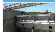
Retarding gates are regulating devices often used downstream of hydroelectric dams to headwater
