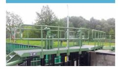
Sluices are engineered structures that make it possible to raise and lower a ship on a barrage to overcome the difference in water levels caused by a dam. A wide variety of different gates are used to close off sluice chambers.
