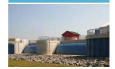
Segment gates are used to precisely control water volumes in the event of high pressures exerted by the impounded water. The principle of load bearing permits operation with minimal positioning forces and consequently low driving power.
